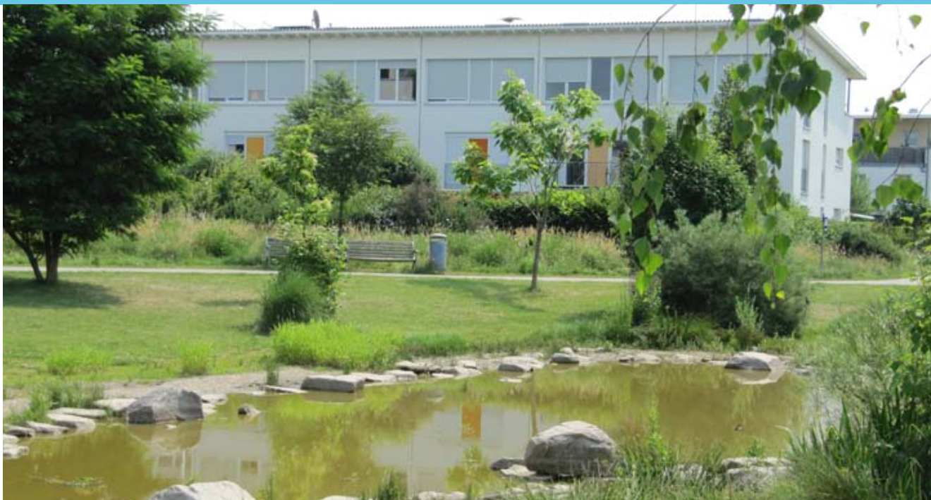
Pond in communal green space as part of the Sustainable Drainage Systems features in Rieselfeld, Freiburg
